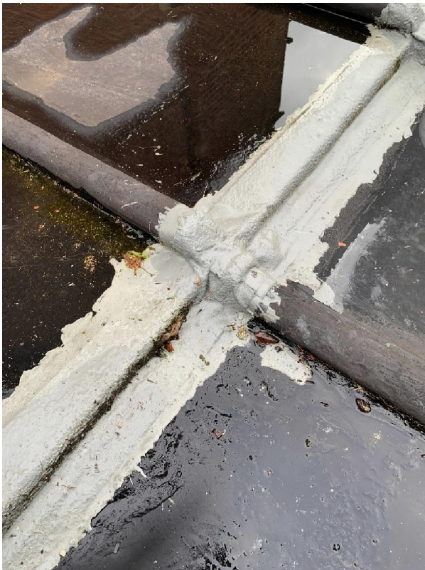
Figure 8 – Detail of above.
