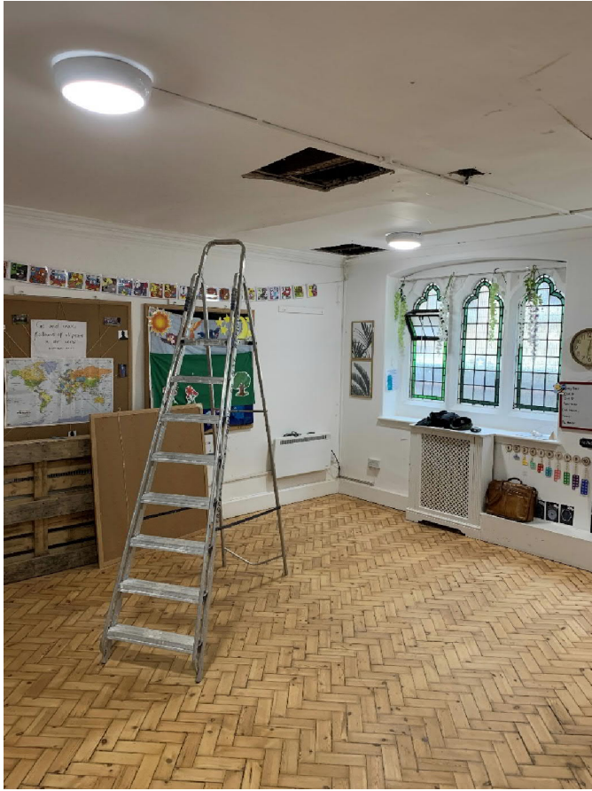
Figure 3 – Vestry showing access opening-up holes.
